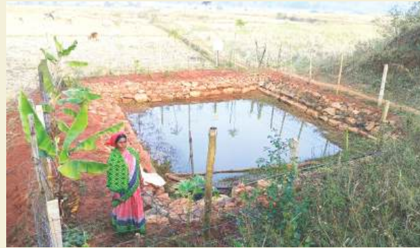
Percolation tank at- Dibari in Sugadabadi GP.
