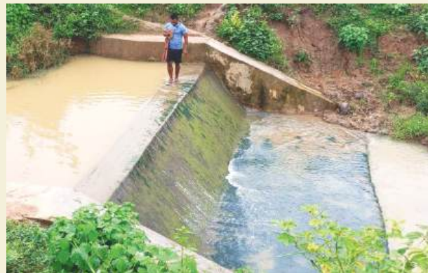
Check dam at-Bierpanga Village in Dadingia GP
