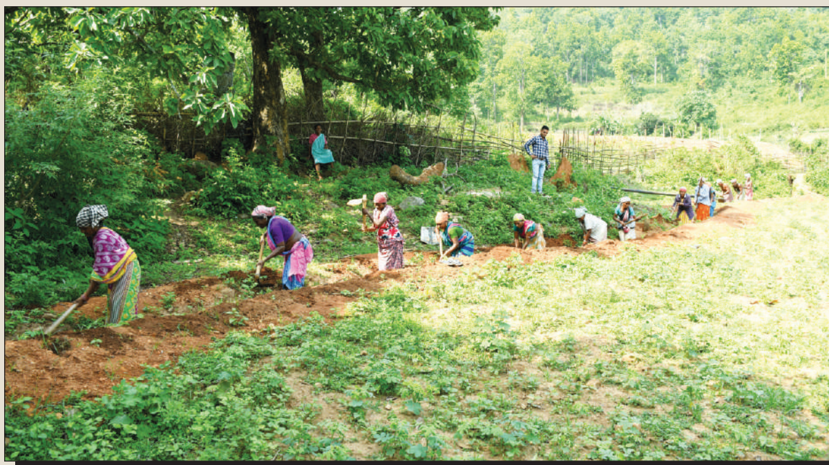
Labour contribution for trench Digging work at DBI site in Penamal Village of Gumamaha G.P
