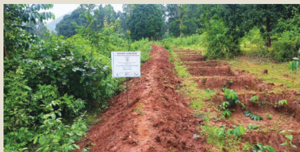
Graded Guided Bund at Musumaha (Gandisi), Dadingia GP, Raikia Block
