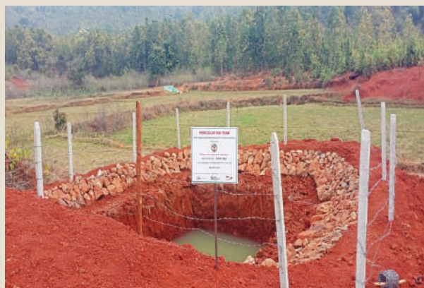
Percolation tank of Ms.Sunita Digal of Bedaguba village Gumamaha GP.
