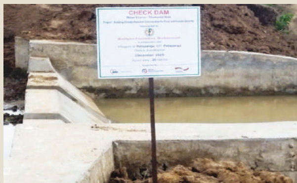
Check Dam-Petapanga Village, Petapanga GP, Raikia Block
