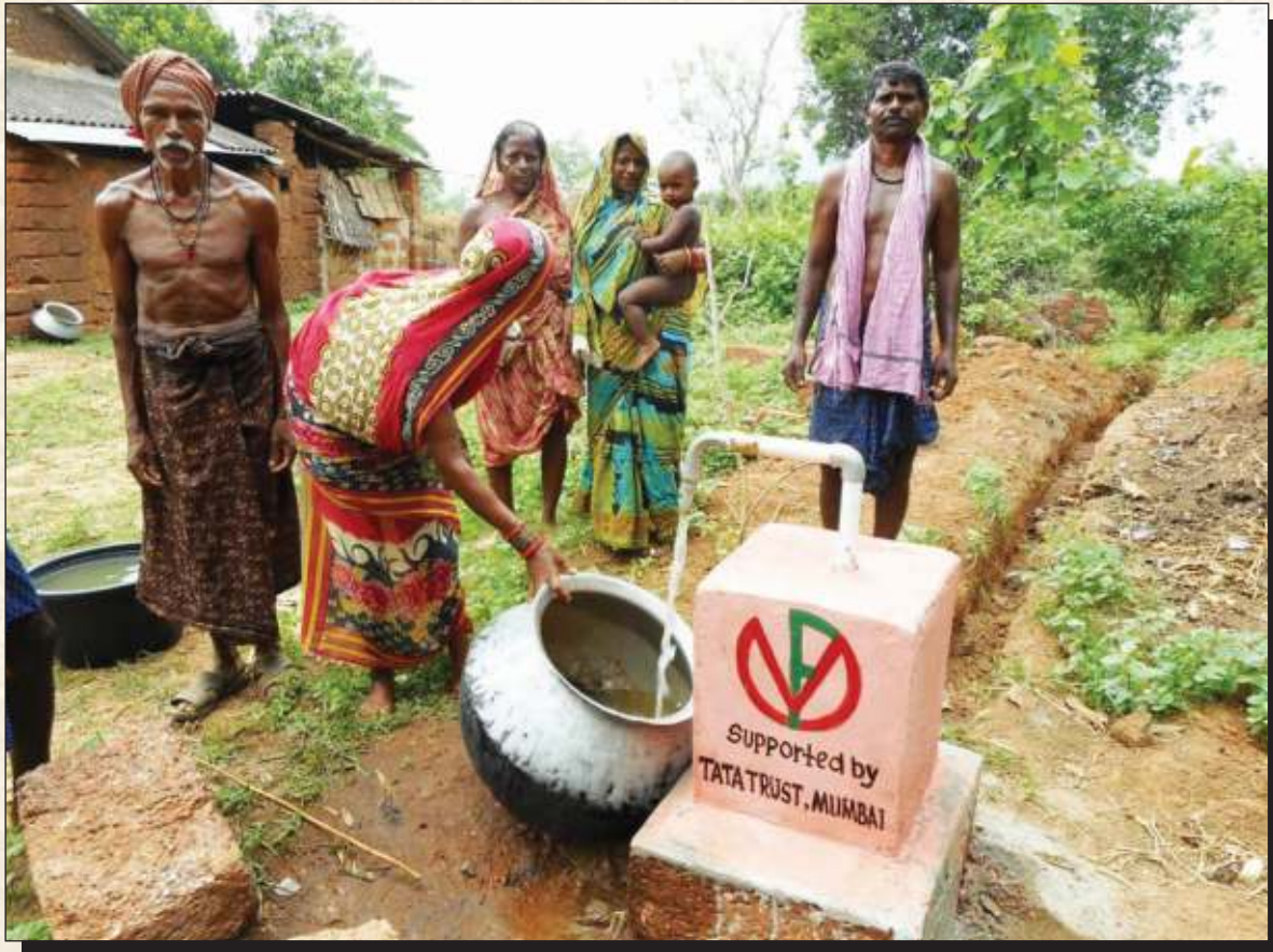
Construction of Riser Assembly for Household water supply
